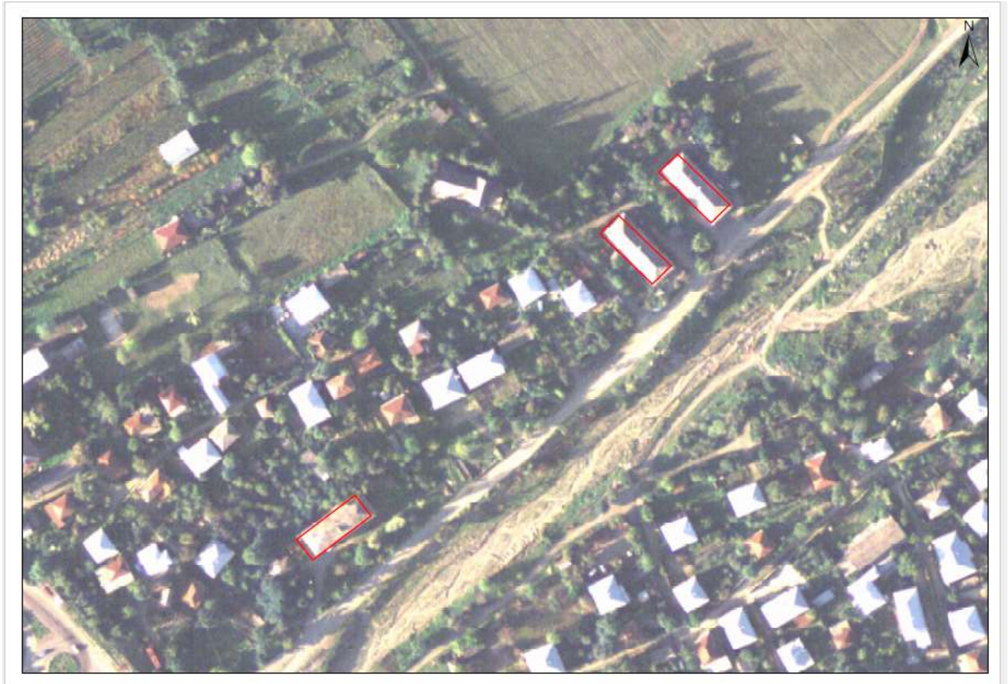
Fig. 2 Project affected houses and 34 Flats from 3 apartment buildings
